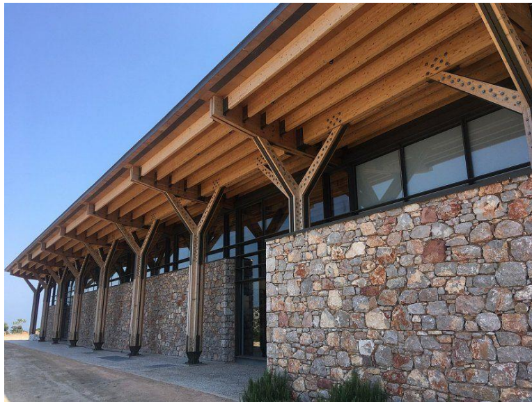
Figure 57. Photograph of area below building eave [Evdemon, Zabulis, 2019].
