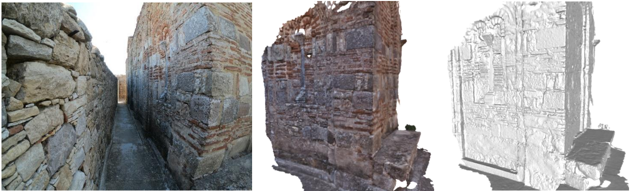
Figure 53. Overview photograph of stone wall and 3D reconstruction [Evdemon, Zabulis, 2019].
